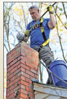
It is recommended to have your chimney swept in the spring, because the deposits are still dry, therefore easier to dislodge. Plus, if the chimney sweep alerts you to a problem, you will also have time to make the necessary repairs before winter.
